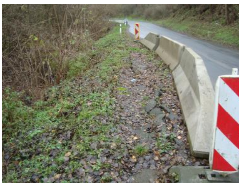
Obr. 08 Sesuv krajnice vozovky, km123,850
