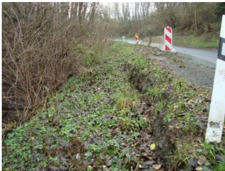
Obr. 07 Sesuv krajnice vozovky, km123,850
